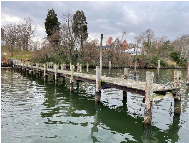
Photo 5 – London Town’s existing 150 LF pier
