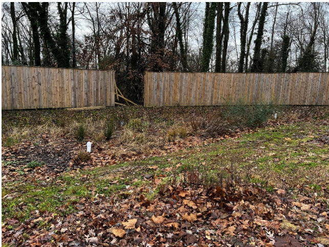
Photo 11 – Existing micro-bioretentation located south of the parking lot
