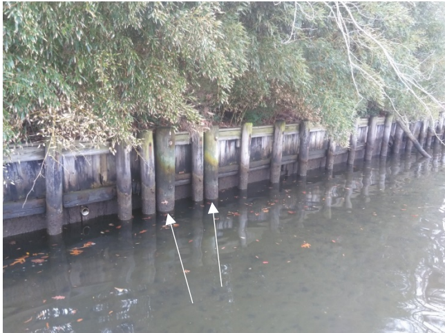
Photo 1 – Added piles along Reach 1 during repair
