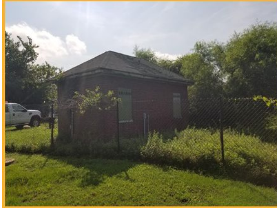
Existing Wastewater Treatment Facility
