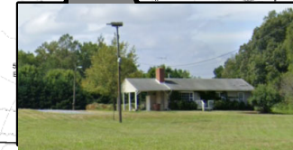
Demolish 1 Story Frame House
