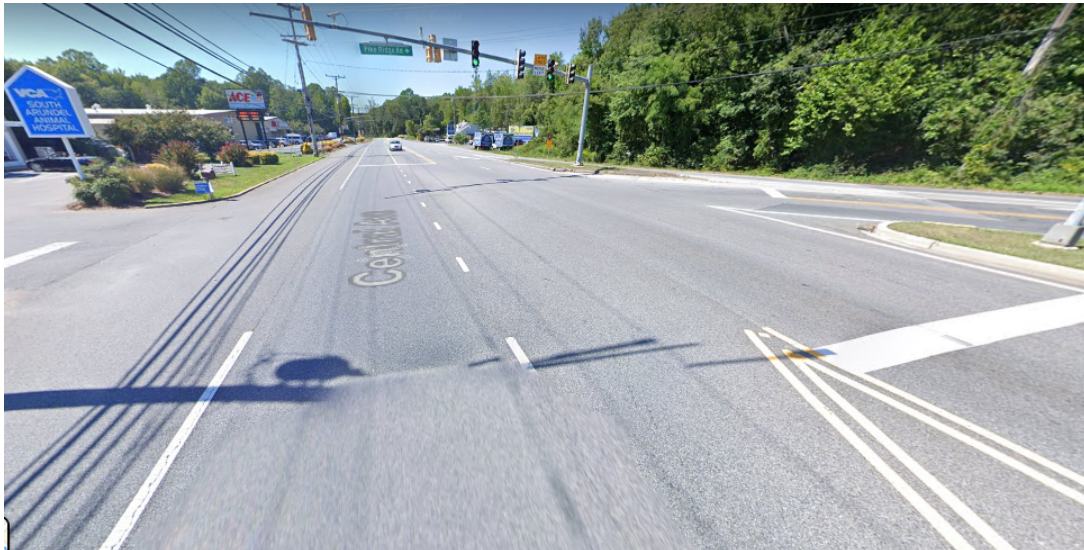
Above: Intersection of Pike Ridge Road and MD 214, multiple driveways and access points in close proximity to intersection and merging.
