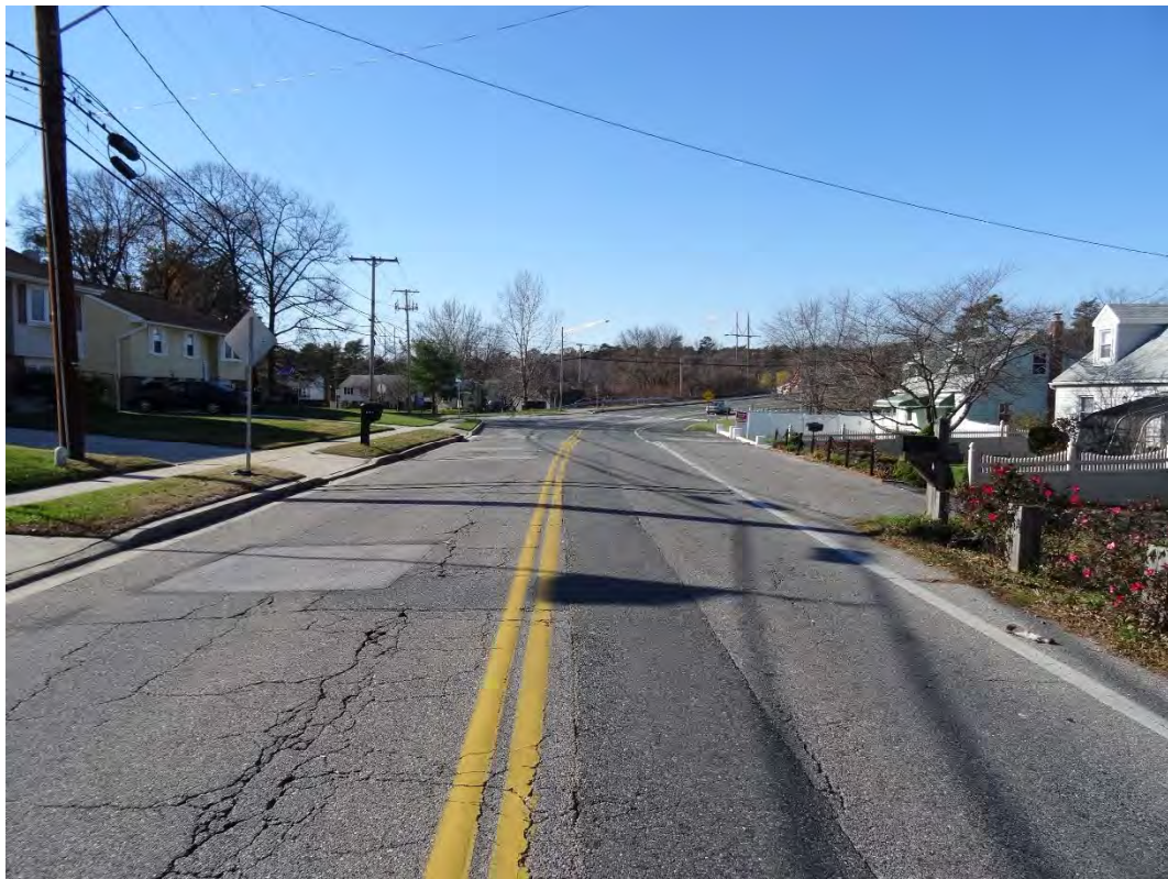
Westbound Stewart Avenue approaching Old Stage Road
