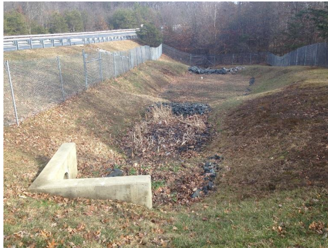
Picture 3: Looking north at SWM facility No. 020108
