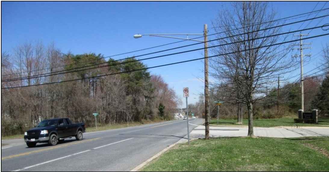
Figure 2 - Utility Pole Impact
