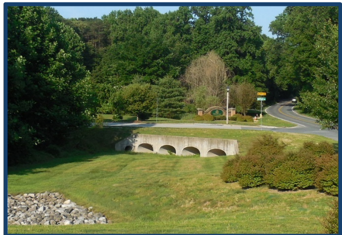
PHOTO 4: LARGE CONCRETE CULVERT AT SUFFOLK WAY
