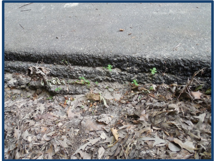
PHOTO 3: EXPOSED PAVEMENT SECTION
