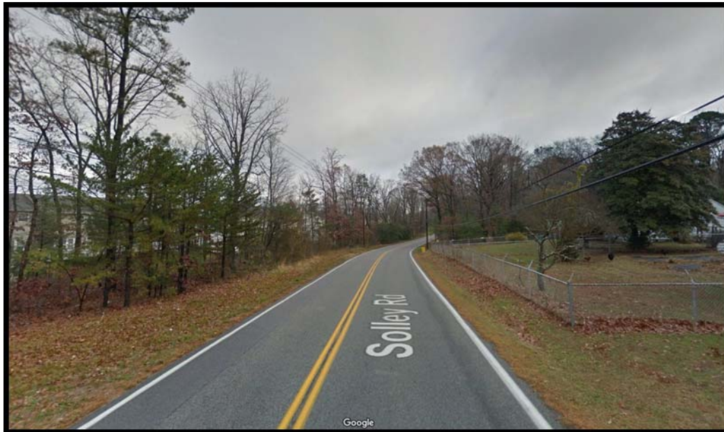
Figure 17: Hot Spot #4, looking north on Solley Road
