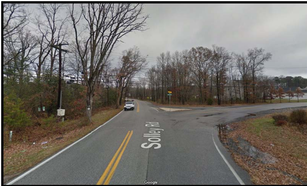
Figure 10: Hot Spot #2, looking north on Solley Road at North Shore Drive
