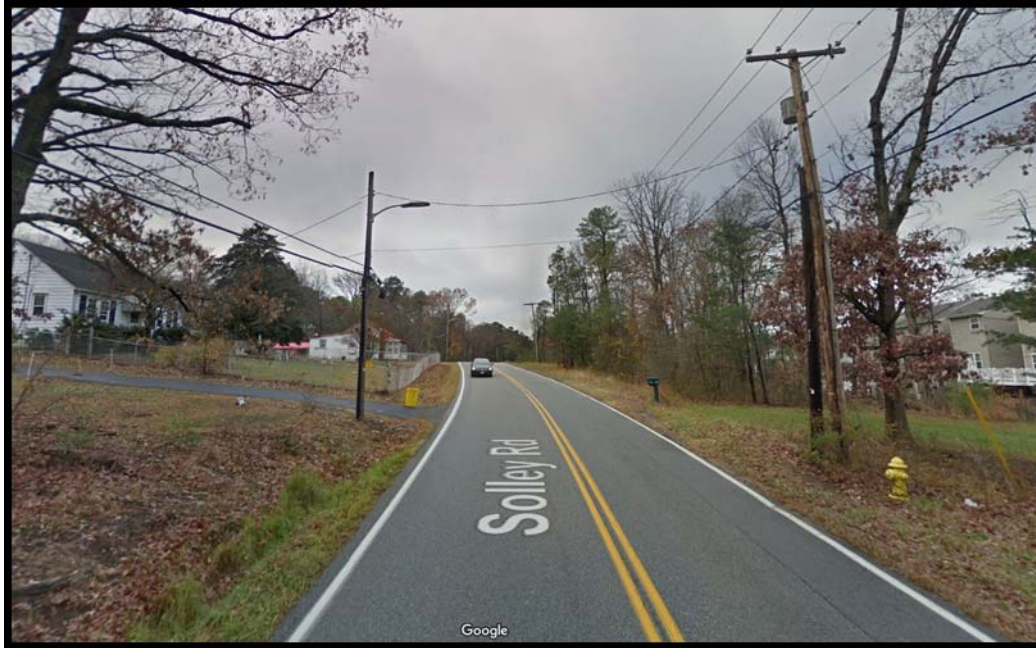
Figure 21: Hot Spot #4, looking south on Solley Road
