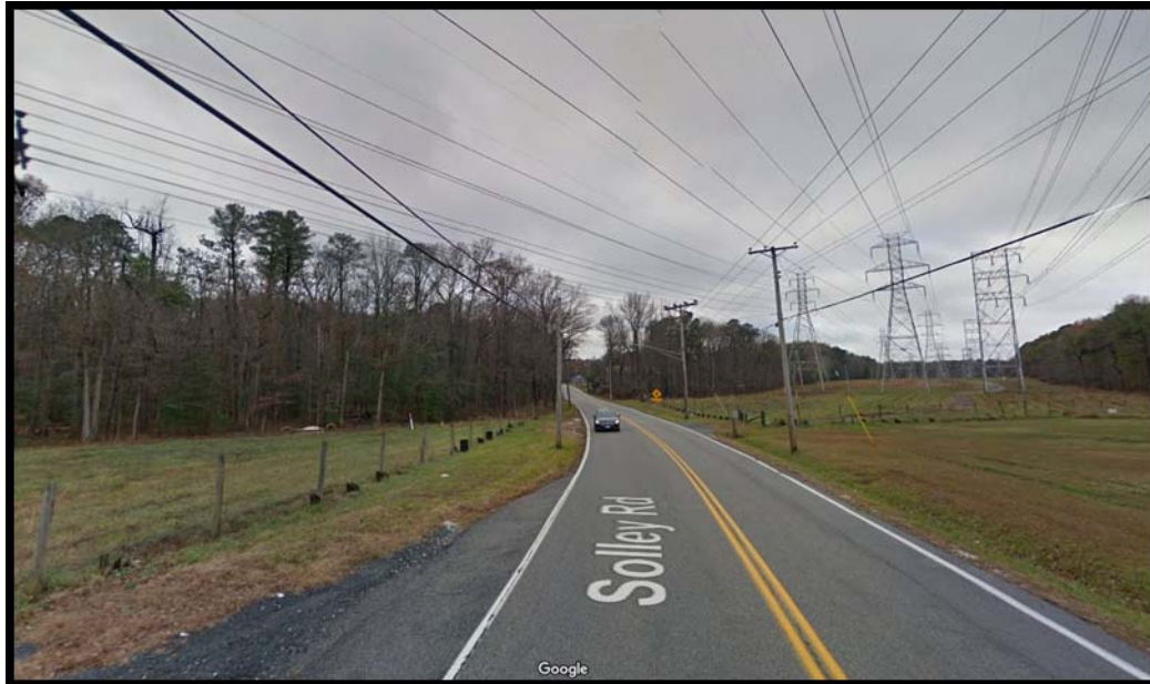
Figure 15: Hot Spot #3, looking south on Solley Road at the power line crossing
