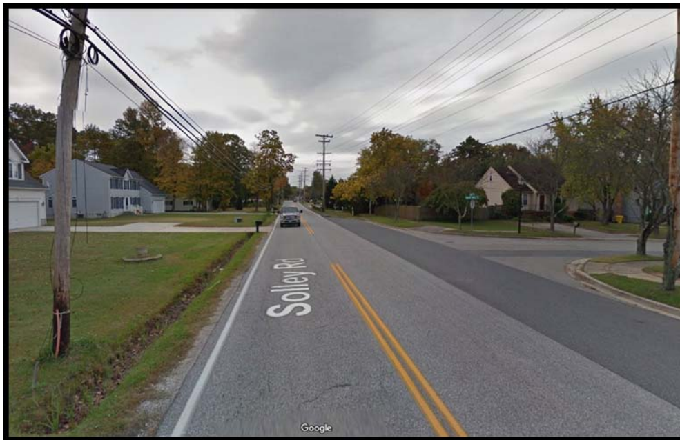
Figure 9: Hot Spot #1, looking south along Solley Road at Nature Walk Lane
