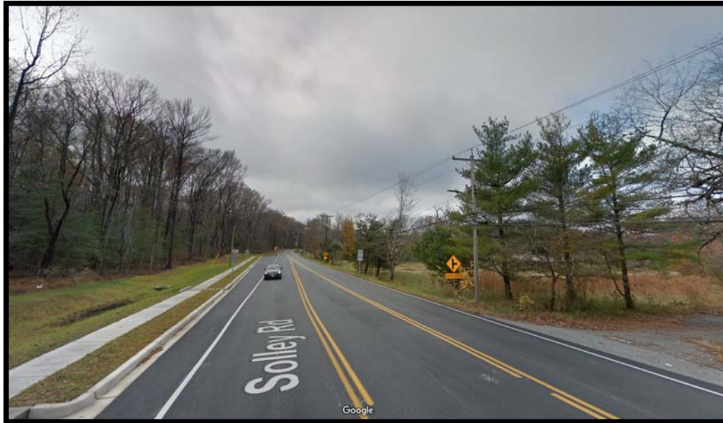
Figure 19: Hot Spot #4, looking south toward Chestnut Springs Lane
