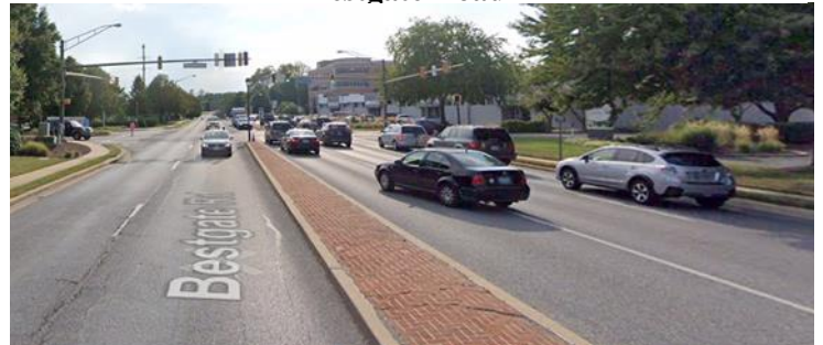
Figure 6: Existing Minor Arterial Roadway – Bestgate Road
