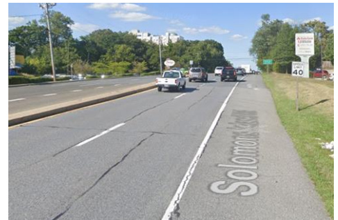
Figure 3: Existing Principal Arterial Roadway - MD 2 (Solomons Island)
