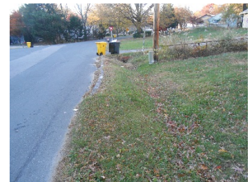
Figure 49 - Existing Ditch West side of Holiday Street - Looking South
