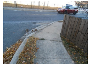
Figure 45 - Existing Pedestrian Ramp - SE Corner of Odenton Road Intersection
