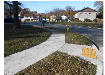
Figure 34 - Existing Ped Ramp to Remain - SW Corner Hammond Lane and Greenwood Street
