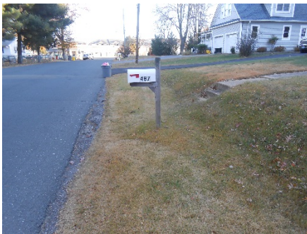
Figure 43 - East Side of Greenwood Looking North - Steep Slope - Retaining Wall Needed
