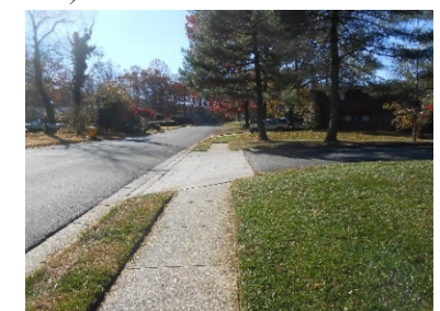
Figure 7 - Higgins Drive - Existing Sidewalk at Church – South End (Looking South)
