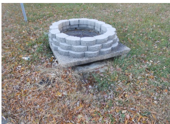
Figure 50 - Existing Yard Inlet - 488 Holiday Street
