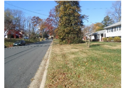
Figure 20 - North Side of Winer Road - Flat Roadside Grading (Typ.) / Possible Tree Removal
