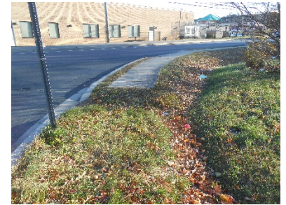
Figure 42 - Existing Sidewalk and Pedestrian Ramp - SE Corner of Odenton Road Intersection
