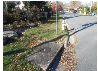
Figure 23 - Utilities at SW Corner of Higgins Drive Intersection
