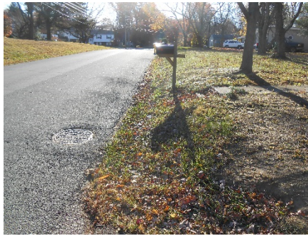
Figure 29 - South Side of Hammond Lane Looking South - Steep Roadside Grading (Typ.)
