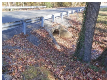
Figure 8 - Existing Culvert at Towsers Branch - East Side of Higgins
