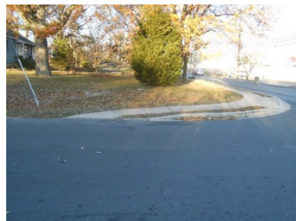
Figure 47 - Existing Pedestrian Ramps - SW Corner of Odenton Road Intersection
