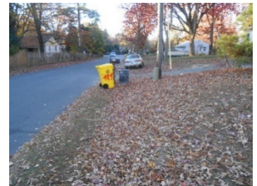
Figure 48 - Steep Roadside Slope - West Side of Holiday Street - Looking South
