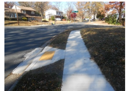
Figure 21 - Existing Pedestrian Ramp - NE Corner Winer Road and Maple Ridge Lane
