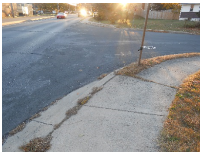
Figure 36 - Existing Pedestrian Ramp - SW Corner of Odenton Road Intersection
