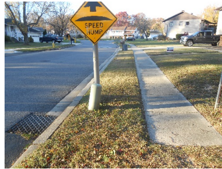
Figure 40 - West Side of Greenwood Street - Tie-in to Existing Sidewalk
