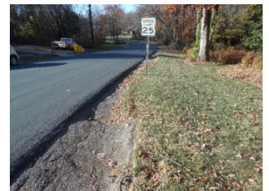
Figure 18 - Existing paved drainage ditch north of Towsers Branch
