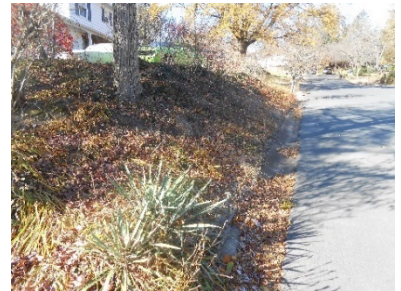
Figure 22 - Steep Grading at 1199 Monie Road
