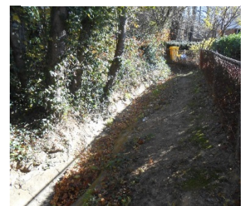
Figure 11 - Concrete Ditch at POI 3
