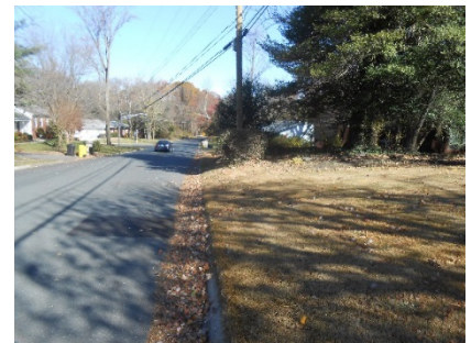
Figure 16 - Retaining Wall at 525 Higgins Drive (Utility Pole)
