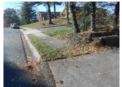
Figure 6 - Higgins Drive - Existing Sidewalk North of church (Looking South)
