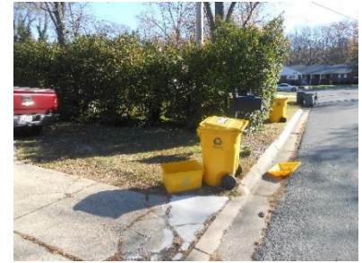
Figure 27 - North Side of Monie Road Looking South - Level Roadside Grading (Typ.) / Shrub Removal
