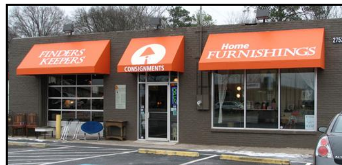
Awnings provide an opportunity to add architectural detail to the façade and enhance the visibility of a business with color and legible signage.
