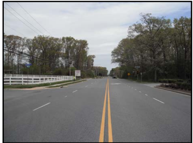
Jumpers Hole Road – North of Benfield Road
