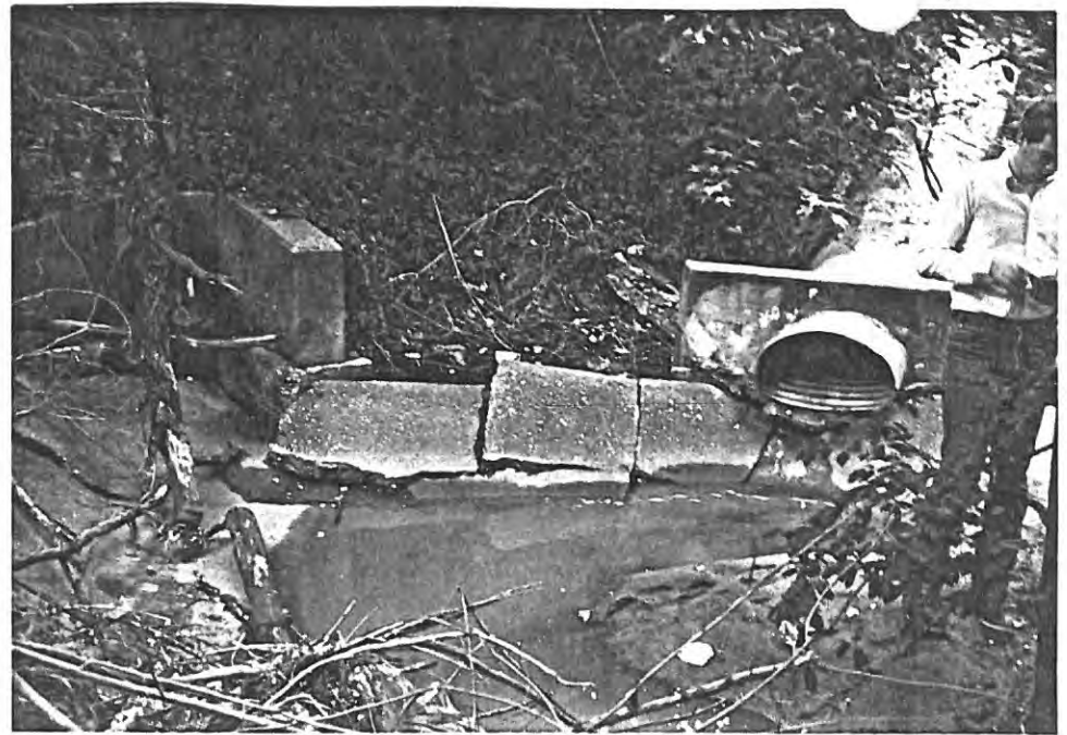
Photo 2 Weems Creek at Outfall of 60" RCP at U.S. Rte. 50 and MD. Rte. 450 Ramps (Pt. B)
