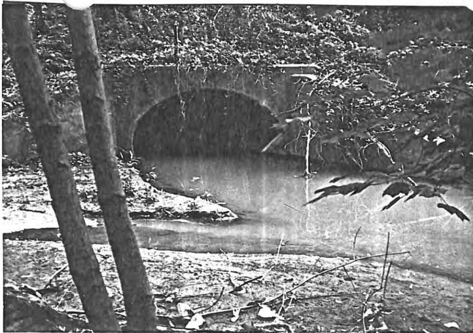
Photo 1 Weems Creek at Outfall of 60" RCP under U.S. Rte. 50 (Pt. A)
