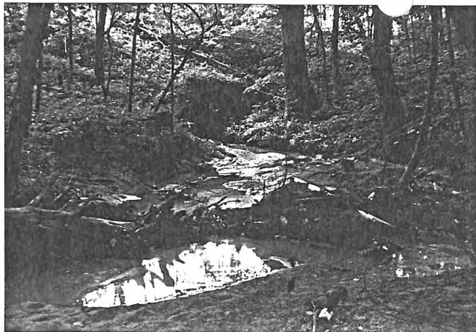
Photo 10 Bank Erosion and Debris on Weems Creek at U.S. Rte. 50 (Pt. J)
