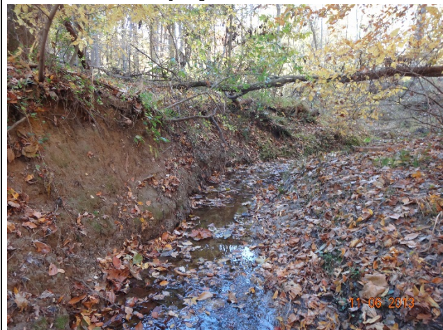
Stream Reach in South Fork Muddy Creek II Subwatershed (RR5) with Degraded Habitat Condition
