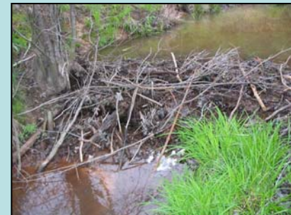
Obstruction with severe impact score located in Patuxent Research Refuge
