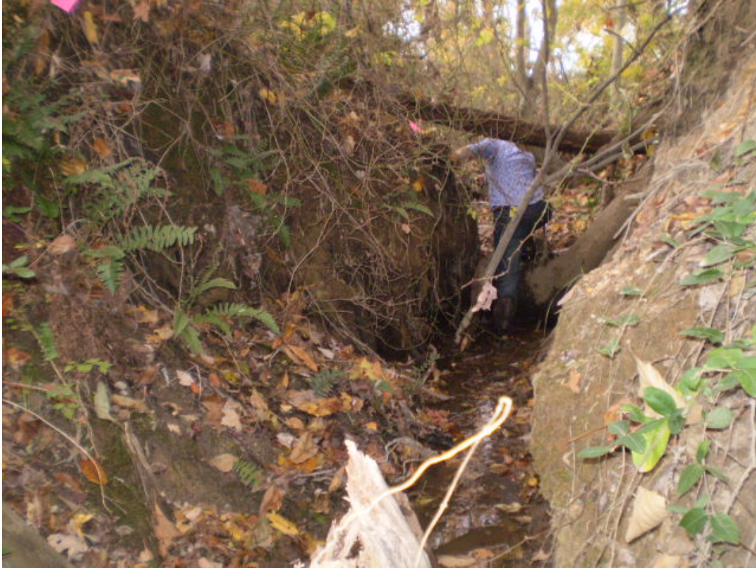
Photo 3. Impaired Reach. View of small headcut looking upstream
