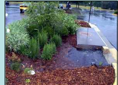
Infiltration practices capture stormwater and allow it to seep into the soil. This rain garden helps capture and filter runoff from a parking lot
