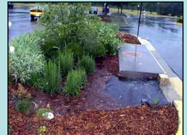
Infiltration practices capture stormwater and allow it to seep into the soil. This rain garden helps capture and filter runoff from a parking lot.
