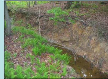
Erosion with moderate impact score located in Patuxent Research Refuge
