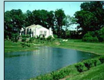
Stormwater detention ponds are wet structures that are often used to capture stormwater runoff in residential areas.
