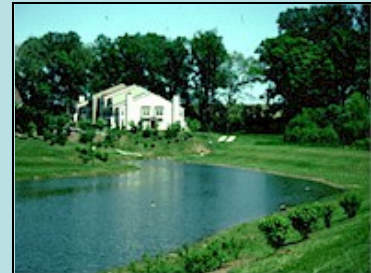
Stormwater detention ponds are wet structures that are often used to capture stormwater runoff in residential areas.
