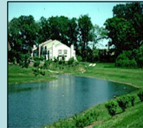
Stormwater detention ponds are wet structures that are often used to capture and detain stormwater runoff from residential and commercial areas.
