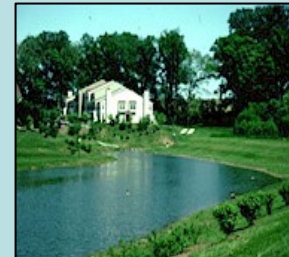
Stormwater detention ponds are wet structures that are often used to capture and detain stormwater runoff from residential and commercial areas.
