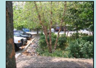
Filtration practices capture stormwater and allow it to seep into a treatment media then infiltrate to the groundwater. This rain garden helps capture and filter runoff from a parking lot.
