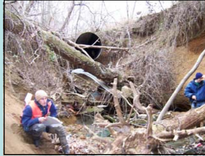
Crossing with extreme impact score located near Riva Road in the vicinity of Riva Drive.
