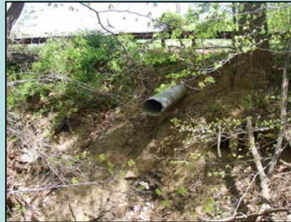
Crossing with extreme impact score located under St. Stephens Church Road.
