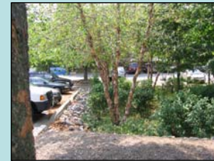
Filtration practices capture stormwater and allow it to seep into a treatment media then infiltrate to the groundwater. This rain garden helps capture and filter runoff from a parking lot.
