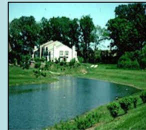
Stormwater detention ponds are wet structures that are often used to capture and detain stormwater runoff from residential and commercial areas.
