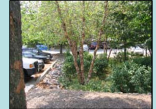
Filtration practices capture stormwater and allow it to seep into a treatment media then infiltrate to the groundwater. This rain garden helps capture and filter runoff from a parking lot.
