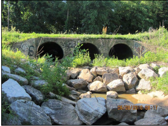
Photo 7 – Triple Barrel Culvert from under Shetlands Lane
