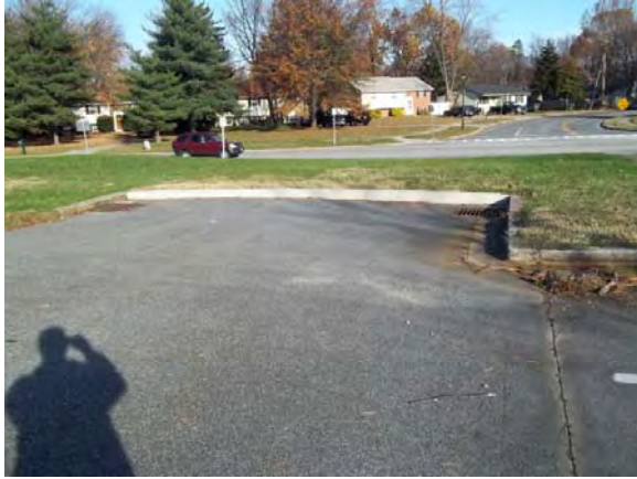
Photo 1 – Location of Storm Inlets, looking north
