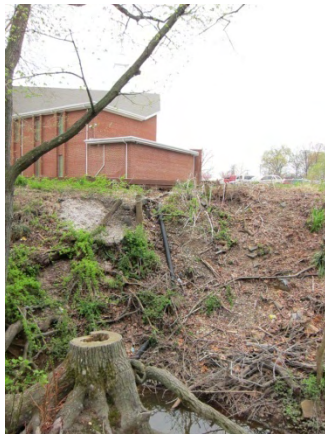
Photo 3 – Stream bank erosion threatening the church parking lot
