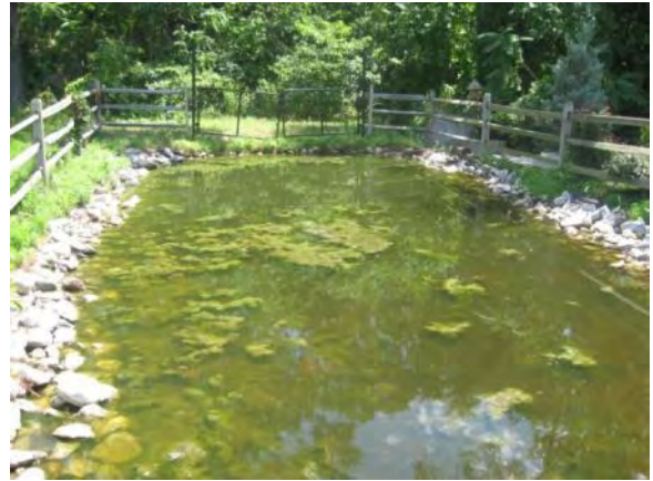
Photo 2 – Existing infiltration BMP at end of 209 th Street filled with water and algae (looking downstream)
