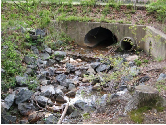
Photo 1 – Three outfall pipes from under Oakwood Drive.
