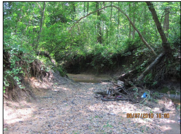
Photo 10 – Continued Severe Bank Erosion at Downstream End of Reach
