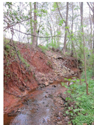
Photo 4 – Stream bank erosion prevalent throughout the Phase 1 restoration area
