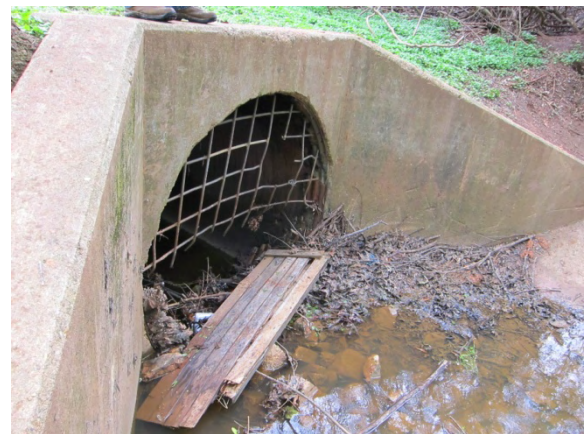
Photo 6 – Inlet where stream returns to piped flow
