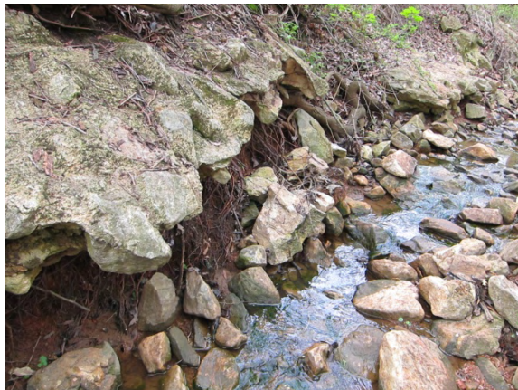
Photo 11 – Cement armoring currently along downstream portion Phase Two.
