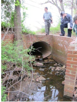
Photo 7 – Outfall from under Funke Road.
