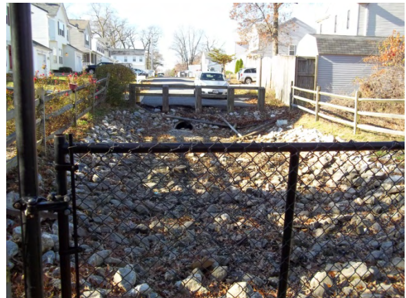
Photo 4 – Existing infiltration BMP (looking upstream)
