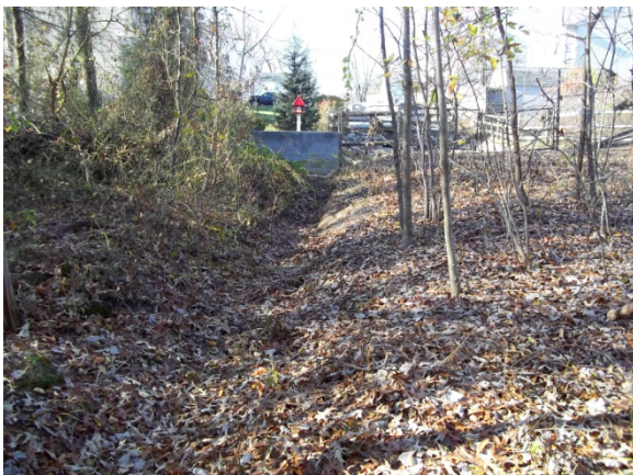
Photo 5 – Opportunistic channel draining infiltration BMP (looking upstream toward BMP)
