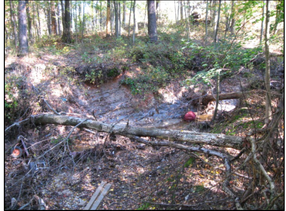
Photo 2 – Severe Bank Erosion in Upstream Portion of Reach
