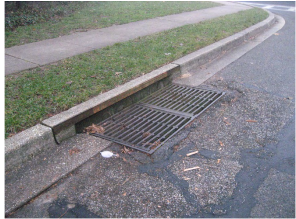
Photo 2 – Catch basin near intersection of Century Towne Road and Shetlands Lane.
