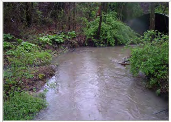
Downstream from Mid-Point
