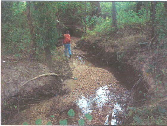
PHOTO 3: DOWNSTREAM END OF SITE AND RTE I-195 CROSSING
