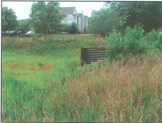
PHOTO 3: EXISTING RISER AND EMBANKMENT
