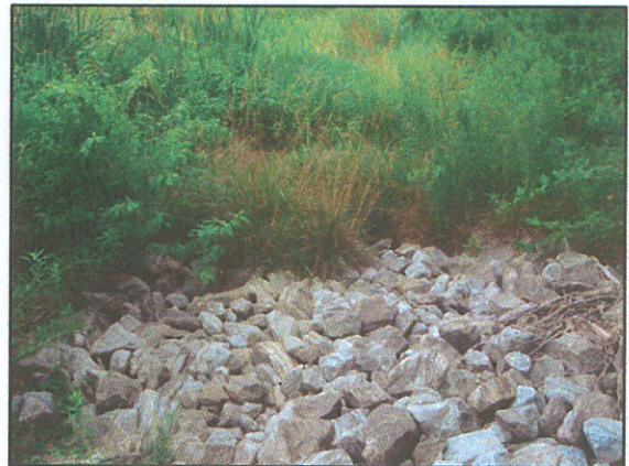
PHOTO 4: EXISTING RIP RAP INFLOW
