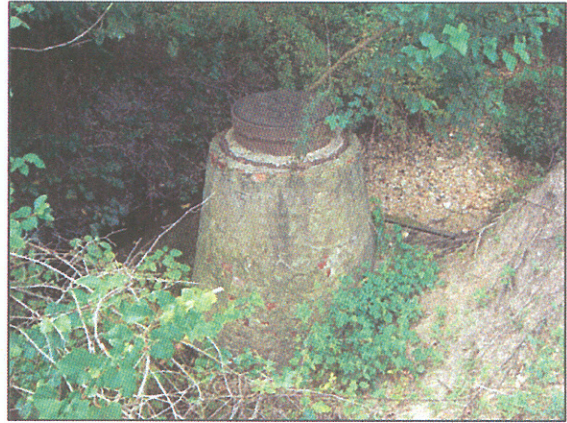
PHOTO 2: VIEW OF EXPOSED SANITARY SEWER STANDPIPE
