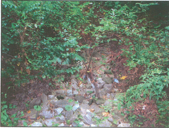
PHOTO 1: UPSTREAM SECTION OF EXISTING RIP RAP CHANNEL
