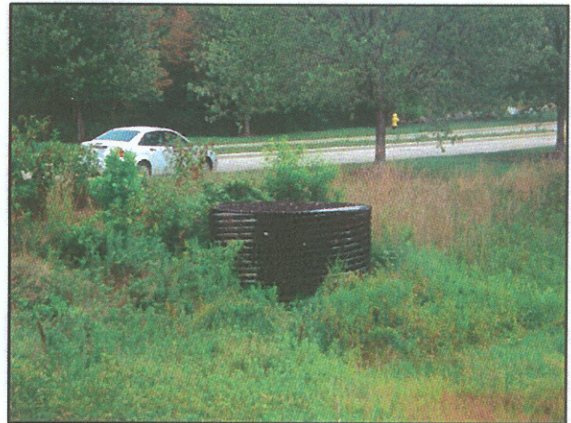
PHOTO 1: EXISTING RISER STRUCTURE
