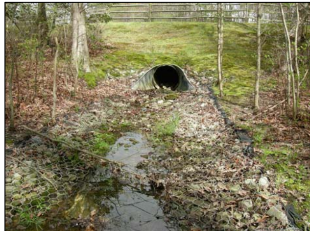
Pipe and Ditch Contributing Flow with Moderate Impact in the Forked Creek Subwatershed (MGL)
