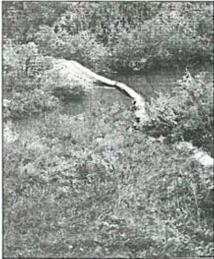
Siltscreen (above) and stormwater management pond (right).
