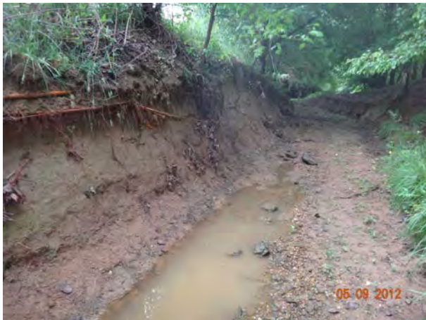
Bank Erosion in the Towsers Branch 2 Subwatershed (LP6) with Moderate Impact Score
