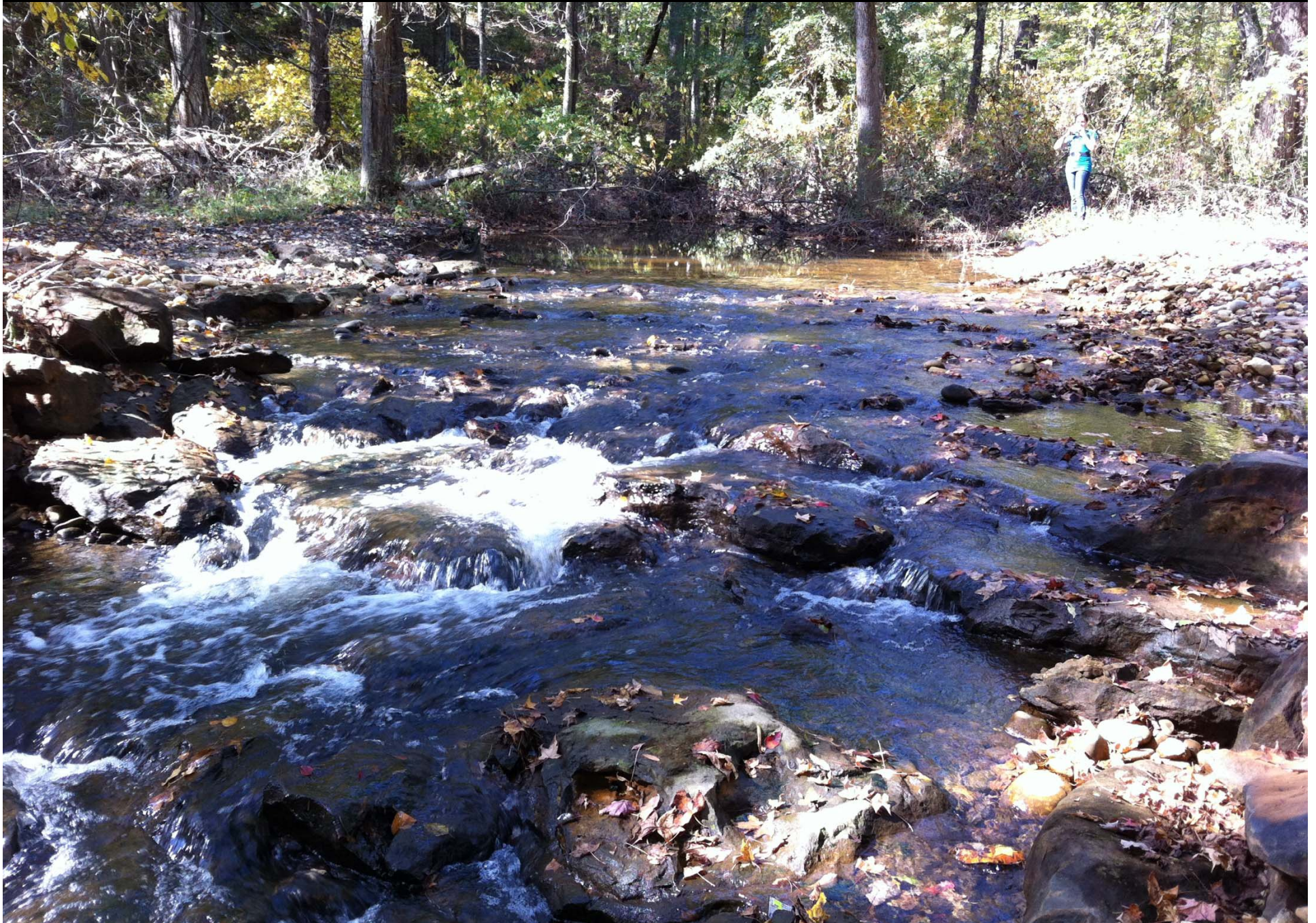
Severn Run Mainstem – After Tropical Storm Lee – Sewer line crossing
