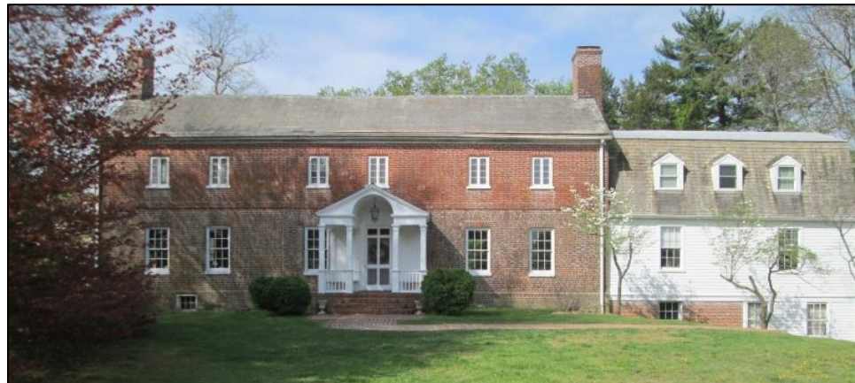
Belvoir Manor (AA-183), constructed in 1736, off of Generals Highway.
