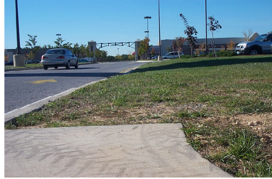
Lack of sidewalk connections on Corridor Rd.
