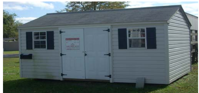
SHEDS LARGER THAN 8 X 8 (64 SQ FT) REQUIRE A BUILDING PERMIT AND POSSIBLY A FOUNDATION
