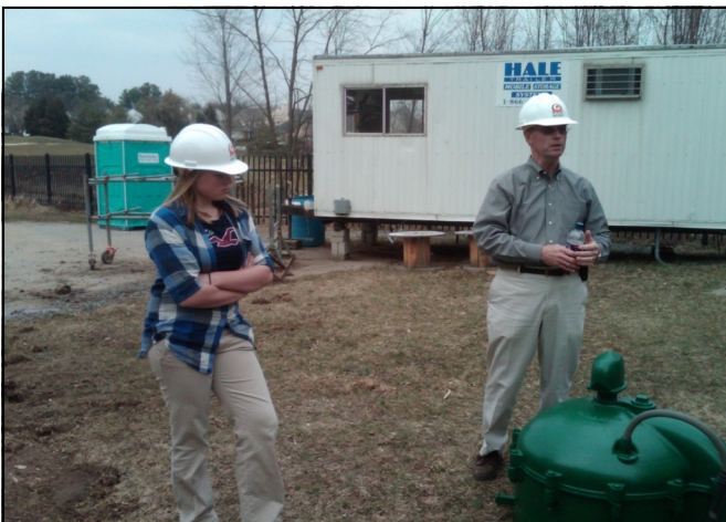
DPW Director Ron Bowen discusses water treatment with Nicole Jackson during a tour of the Crofton Meadows II Water Treatment Facility.
