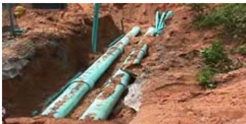
Water line exposed in preparation for maintenance.
