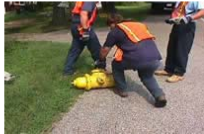
Workers repair a fire hydrant struck by a vehicle.
