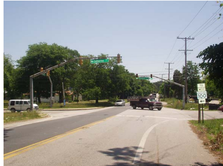
MD 648 (north of intersection) looking toward Magothy Bridge Road
