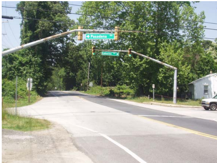
MD 648 (south of intersection) looking toward MD 177 (Mountain Road)
