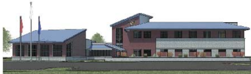
South Elevation From Pasadena Road
