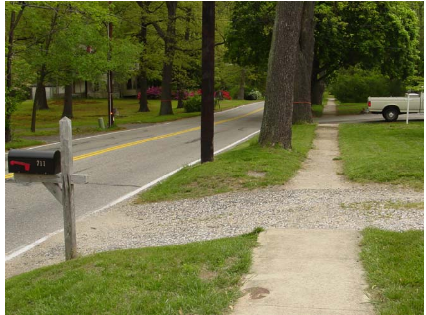
EXISTING DETERIORATED DRIVEWAY APRON ALONG PASADENA ROAD #711 PASADENA ROAD
