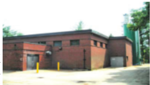
Severndale Water Treatment Plant
