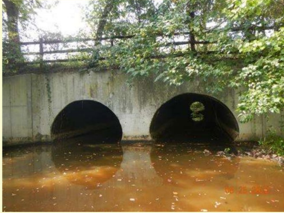
BRIDGE NO. AA4020001 TOWN CENTER BLVD. OVER TRIBUTARY TO SEVERN RUN
