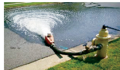
A water line is being flushed to clean out any sediment that has built up over time. This is part of the routine maintenance that Anne Arundel County performs to keep the water distribution system functioning at its highest level.
