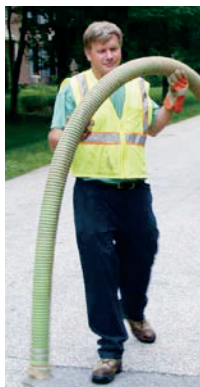
Employees work to repair a water line.
