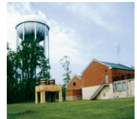
Crofton Meadows Water Treatment Plant
