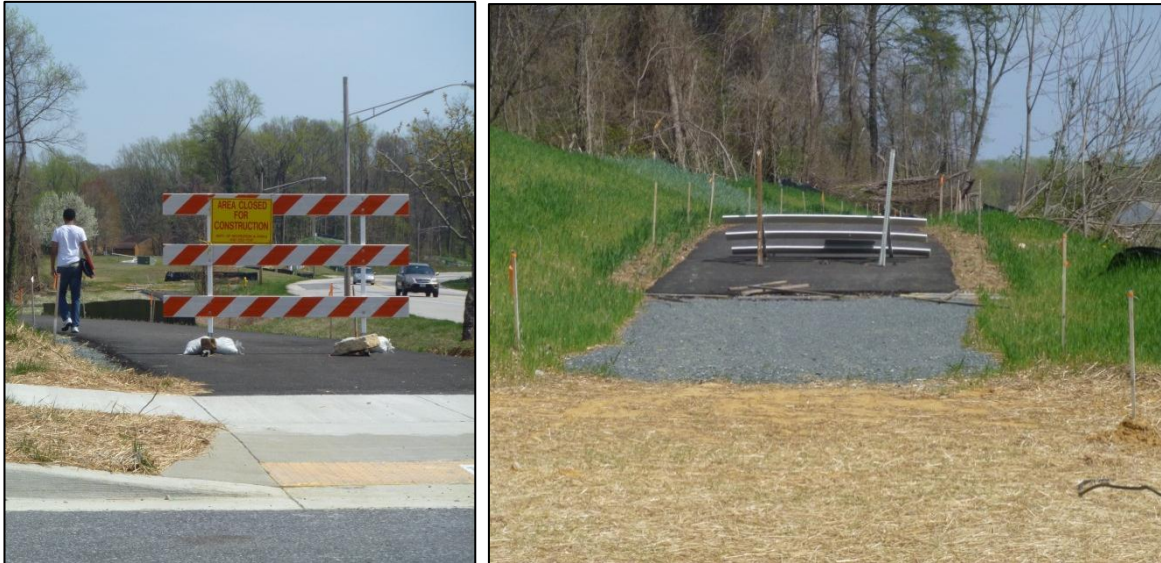
Broadneck Trail Phase IA under construction in April 2013.
