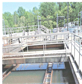
Arnold Sedimentation Basin
